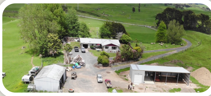
Wharekiri Managers House and New Implement Shed
